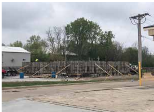
Trenton’s official branch location is located just to the west of its temporary home and was slated for completion in the fall of 2019. Full-service banking will continue in the permanent space near the intersection of Highway 65 and Highway 6.
